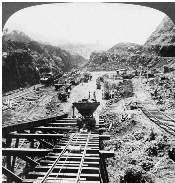
Above: The construction of the Panama Canal.
